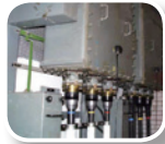
Power sensitive equipment
